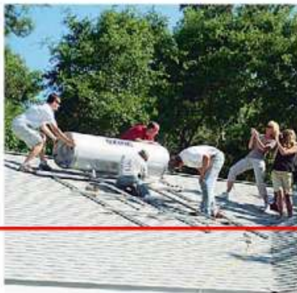
Installation of a drain-back system in Tallahassee, Florida
